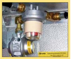
**Option 2** Loosen and rotate the pre fitted elbow 30 degrees -Fit an 01-1755 automatic changeover head. Notice we have used a 01-1677 on the right outlet due to the restriction of the back wall
