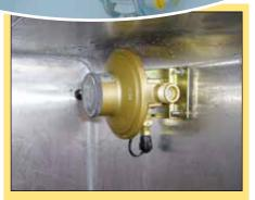
**Typical configuration with** Regulator in top right and inlet facing you.
