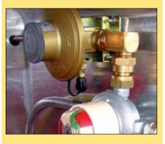
Option 2 Fit an 01-1755 automatic changeover head using a 01-1677 right angled adaptor. Height has been lowered so use Stainless Steel 01-6050-SS.
